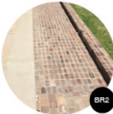
BR1 RECYCLED BRICK BITS PAVING BELOW DRIP LINES
